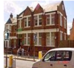
CHC's existing building— soon to make way for ...see story
